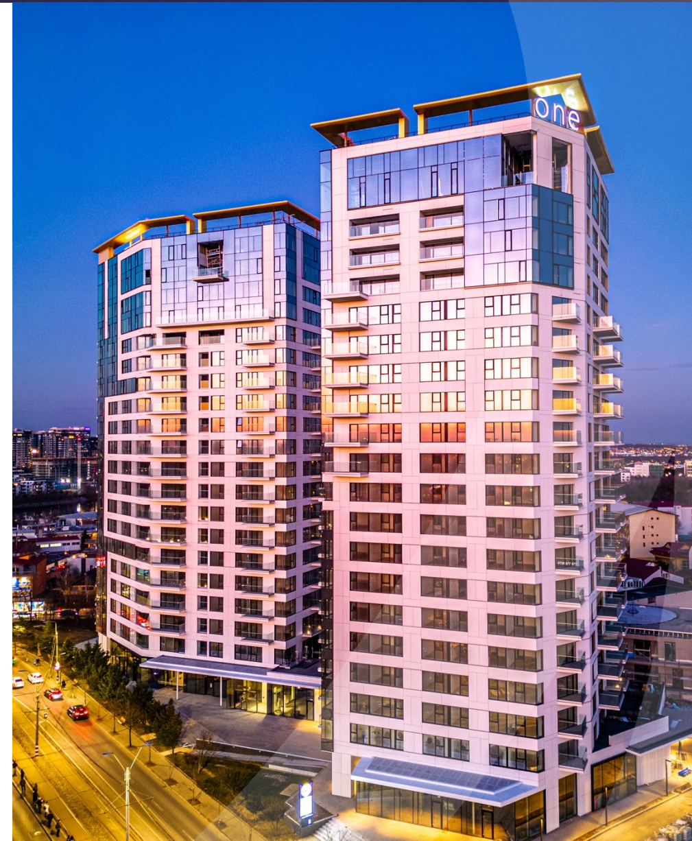
One Verdi Park , the tallest residential towers in northern Bucharest, delivered in 2023.
